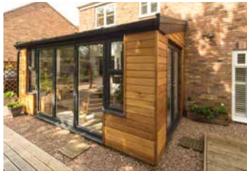
Horizontal Timber Boards
