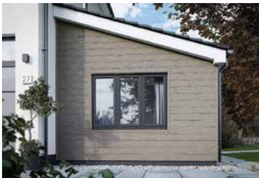
Horizontal Cement Boards
