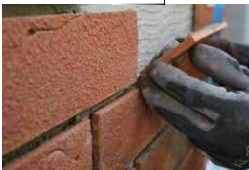
Brick Slips Application
