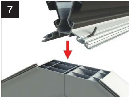
7 Place and support the ridge, ensuring it is central to the gable frame.
