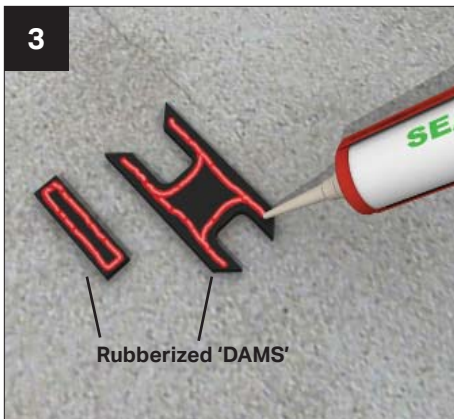
3 Take 'rubberized' sealer strips and generously butter with silicone.
