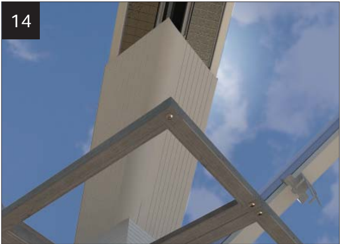
Measure and fit the standard valley undercladding NVU-V between the eaves and mark 'C'. Scribe to suit.
